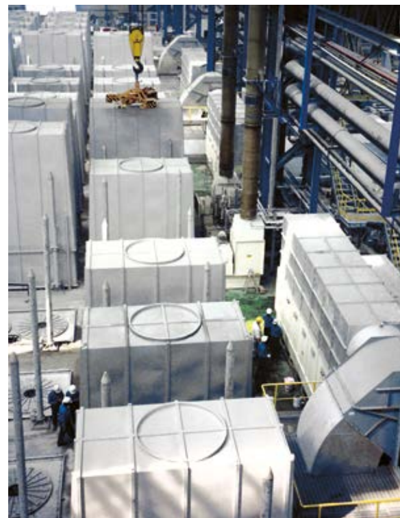
▲ Coil Cooling and Storage Units (CCSU) offering final cooling with dried air
